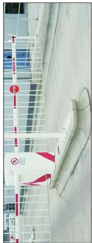
HIGH CONTAINMENT CURB 1500MM FROM EDGE
